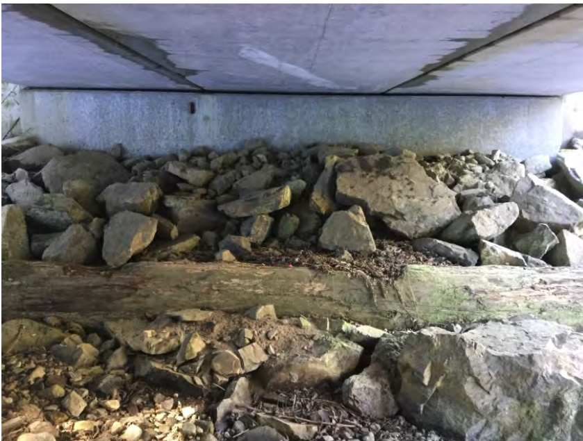
Left Bank Abutment when facing downstream
