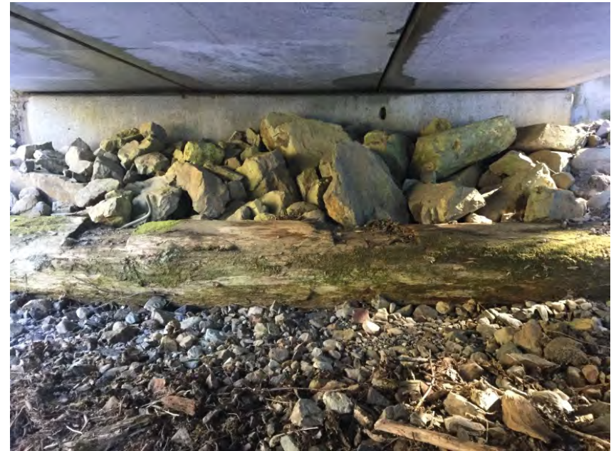
Right Bank Abutment when facing downstream
