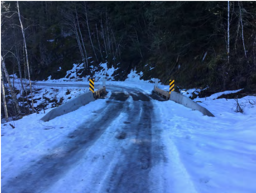
Approach from Left Bank when facing downstream
